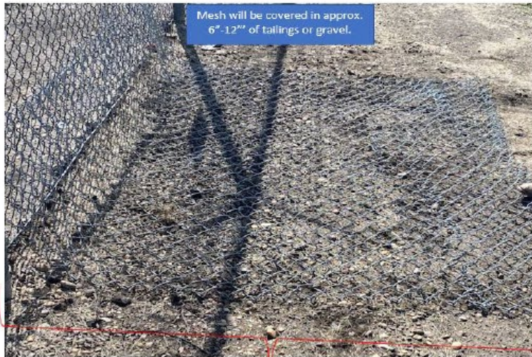
Approx. 4" coverage with gravel or asphalt tailings
